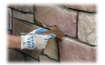
Never use water to clean wet mortar because it will coat the stone with a foggy layer of mortar. Unlike brick and real stone, cast stone cannot be washed with acid. Also, don't power-wash the stone because high pressure may damage the surface.
