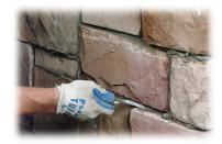
Use a strike tool to pack and remove excess mortar. Again, you must ensure that water is unable to penetrate the mortar joints. If any holes or voids are apparent, pack or fill them with mortar. After the joints are worked to the appropriate depth, use a wisk broom or automotive parts brush to clean and buff the joints.
